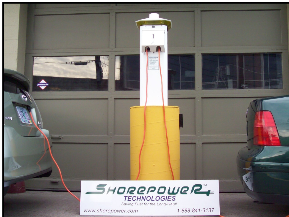
Truck Stop Electrification Pedestals
