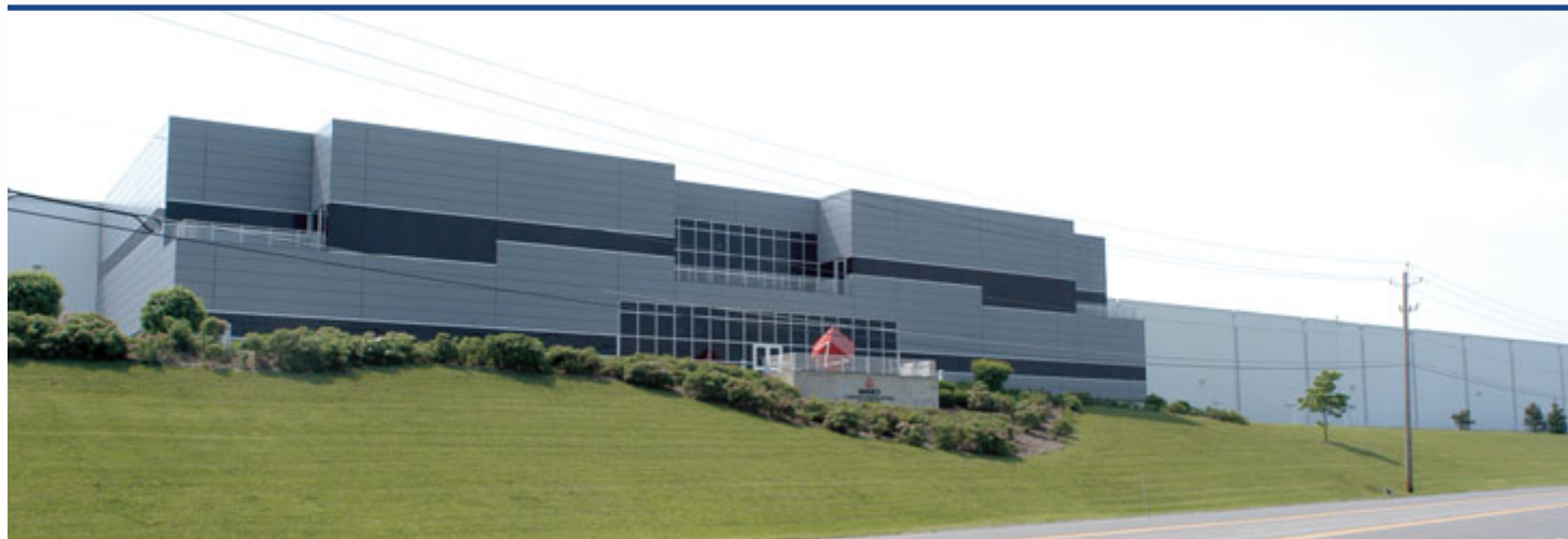
Maines’ flagship distribution center in Conklin, N.Y
